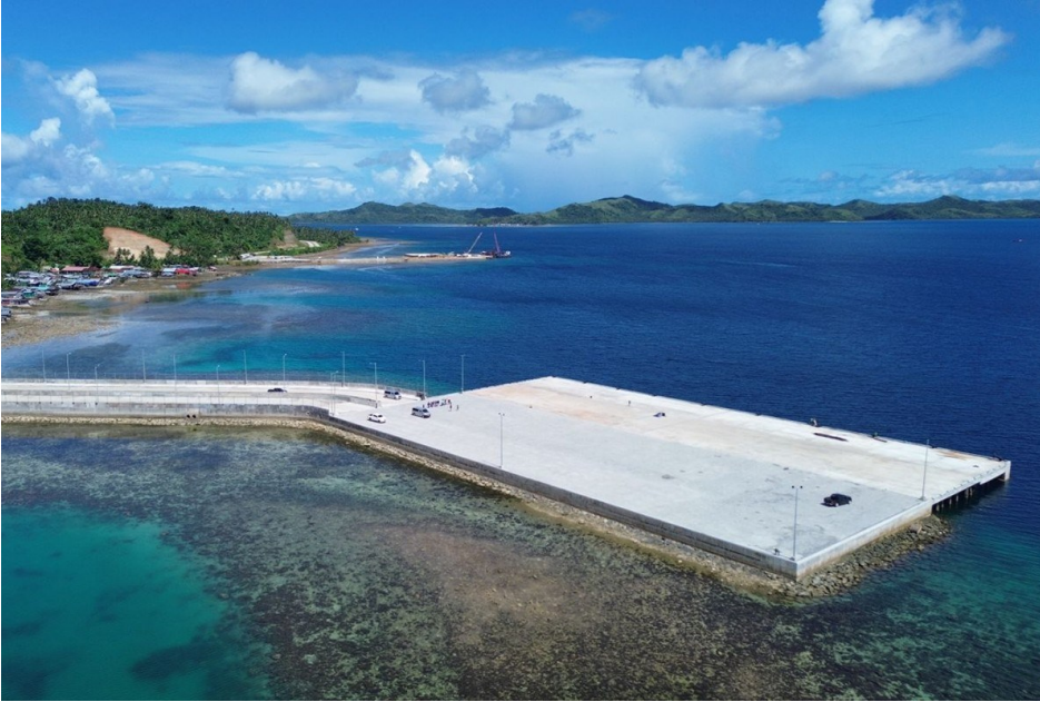
The Jubang Cruise Port in Dapa, Siargao Islands, Surigao Del Norte. (Photo courtesy: MAC Builders Corporation)
